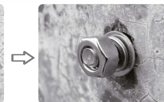
3. Place the expansion screw into the hole.
