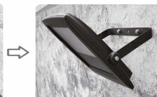
8. Install the flood light and adjust the light direction as needed. Tighten the fixings.
