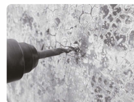
1. Measure the holes from the light bracket and make two marks to drill.
